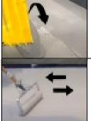
**Cut in edges and stem walls** if applicable with 4" Chip Brush and **pour a band** of mixed material out onto the floor roughly 6-8" wide
