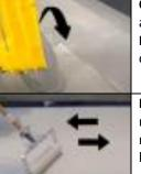
**Cut in edges and stem walls** if applicable with 4" chip brush and **Pour a band** of mixed material out onto the floor roughly 6-8" wide
