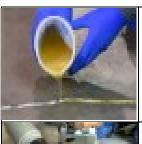
Pour material into prepped and cleaned cracks and spalls. Slightly overfill substrate defects and allow to dry 15-20 mins.
