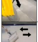
**Cut in edges and stem walls** if applicable with 4" chip brush and **Pour a band** of mixed material out onto the floor roughly 6-8" wide
