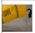
Pour a band of mixed material out onto the floor roughly 6-8" wide. Begin by cutting-in the concrete stem walls and around the edges with a chip brush or weenie roller. Always keeping a wet edge, do not work more than 15-20 min ahead of main body of the floor.
